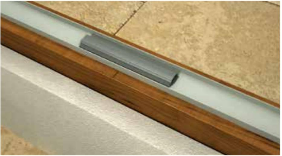
**5.** Insert the SC spacing profile on the top of the glass element.
