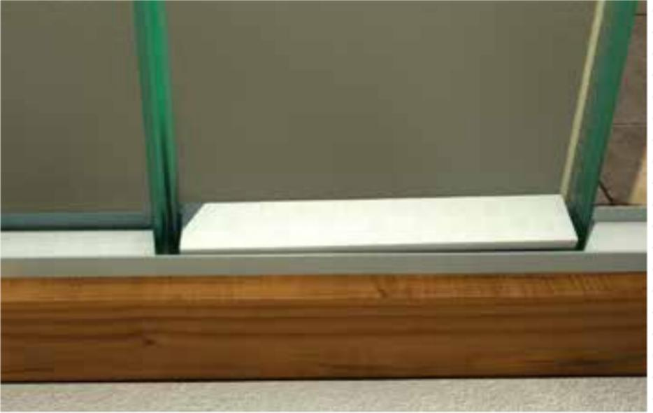
**8.** You have 2 more sheets left on each side. Start with the one at the end. The remaining space is not enough for both sheets to fit. Measure the existing space first and then cut the last glass element vertically, so that the one you set next to it will perfectly fit.
