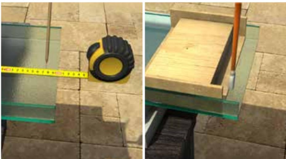
**3.** Measure the horizontal distance of the span where the U-GLAS will be placed. Mark the halfway point - from here you will start to install simultaneously the glass elements to the right and to the left.
