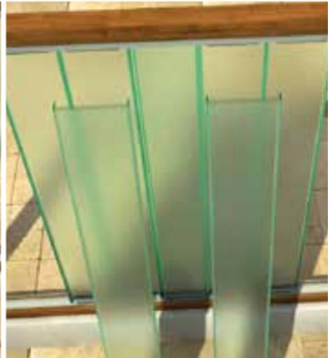
**9.** You have 2 more sheets left on each side. Start with the one at the end. The remaining space is not enough for both sheets to fit. Measure the existing space first and then cut the last glass sheet vertically, so that the one you set next to it will perfectly fit.
